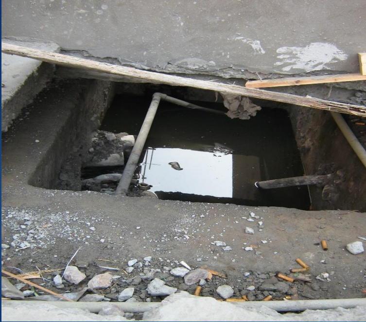
Unsealed plumbing in factory, cigarette butts & stick in glue pot for direct contact.
